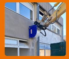
While renovating of a primary school building in Giessen, contracting company Leinweber used a large excavator and a KEMROC EX 60 HD surface milling attachment.
