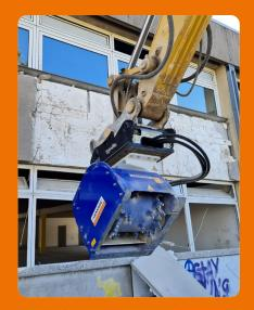
Thanks to depth control, which can be adjusted to the nearest millimeter, it was possible to remove the concrete outer shell from the insulation layer and dispose of the milled material.
