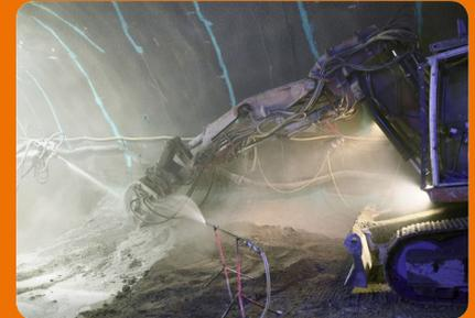
BeMo used a KEMROC cutter wheel to separate the floor of the crown in the South Branch of the light rail tunnel to eliminate noise and vibration when using a breaker.
