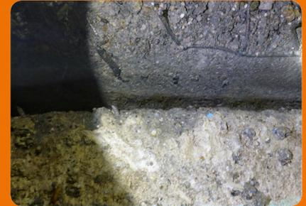
The KEMROC cutter wheel went through the 50 cm thick, reinforced concrete base in the crown section to the bedrock below.
