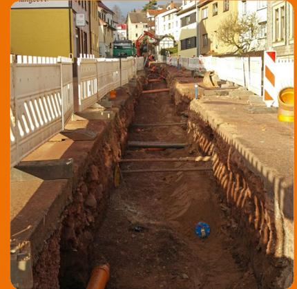
AIT had to excavate trenches and lay pipes in hard sandstone at Finsterbergen. Renovation work along Rennsteigstrasse is due for completion by the end of 2017.
