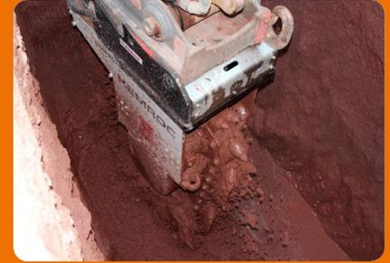
At times, the chain cutter had to work in very abrasive sandstone mud. According to the operator, wear rates remained at acceptable levels.
