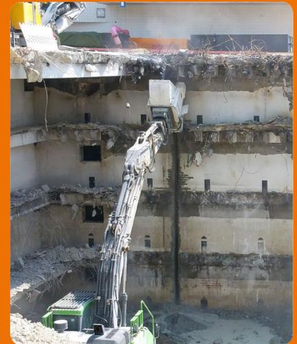
The demolition and foundations specialist company Prünstner uses a KEMROC ERW 220 cutter wheel to demolish an underground parking garage.
