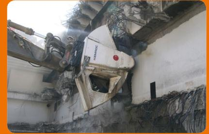
At rapid speed, the KEMROC cutter wheel cutting through heavily re-enforced concrete walls and the bored piles located behind them.
