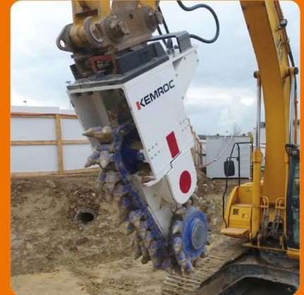
Construction company Gubler using a KEMROC chain cutter on a 22 ton excavator at a job site in Mettmenstetten near Zurich.
