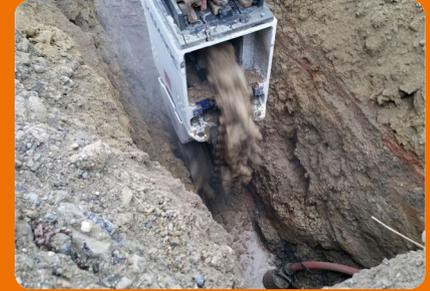
An additional advantage from using a grinder: the extracted material has a fine grain size and can be used straight away as fill material resulting in lower transport costs and savings on fill material.
