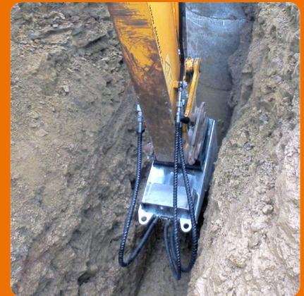
Trenches with depths of around 5 m could be excavated with near vertical side walls. This resulted in significant savings in transport cost and fill material.
