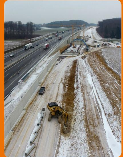
In hard limestone, the STUTZ/BUNTE consortium used hydraulic excavators with KEMROC chain cutters to excavate trenches that will be carrying power cables on the Wendlingen – Ulm section of the high-speed train line being constructed.
