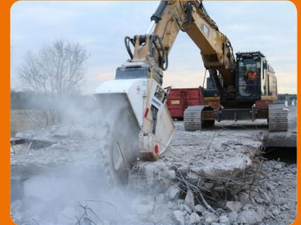
To demolish the eastern half of the Düte bridge near Osnabrück, the demolition company UPEK used a KEMROC DMW 220 cutter wheel for the sensitive work of cutting the bridge deck.
