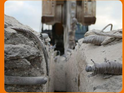
Even in the tough concrete, filled with re-enforcement and tension bars, the cutter wheel achieved a demolition rate of one meter of road length per hour.
