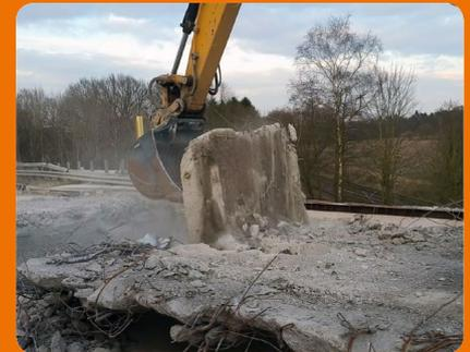
One square meter segments were cut out of the concrete bridge deck, pulled over onto the remaining decking and then broken down using traditional excavator attachments.
