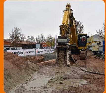
After about two hours of set-up time work can start on the construction of soil-cement structures. In practice, productivity rates of one meter per minute have been achieved.
