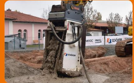
The binder suspension is fed through a hose to the injectors located on the sides. The composition of the binder material injected determines the density and strength of the soil-cement structure.
