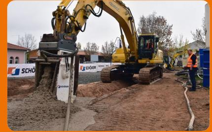
Soil stabilisation by mixing soil and cement while injecting a binder suspension – with the new SCHÖKEM process there is no transportation of soil, it is all done in-situ.
