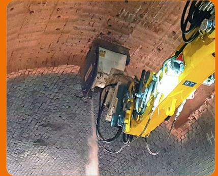
EX planers can be used to work overhead. But to orientate the patch planer correctly in the narrow Hasselborner Tunnel, a tiltrotator had to be used.
