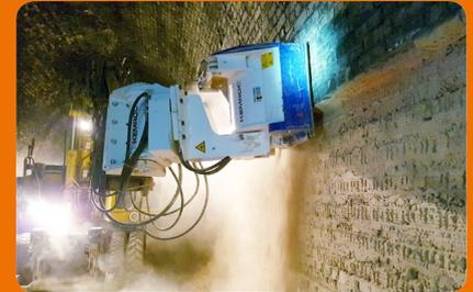
Where required, the KEMROC EX 45 HD was used to remove a 25 – 30 cm deep layer from the brick tunnel lining in the crown of the tunnel.
