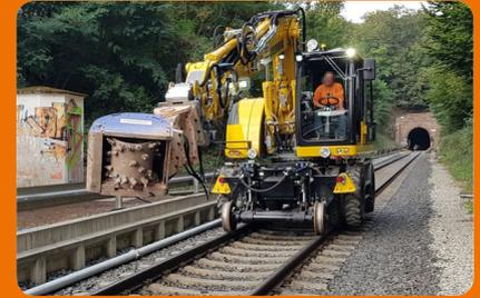
At the Hasselborner tunnel renovation project in central Hessen, Baresel used a KEMROC patch planer mounted on a railway excavator.
