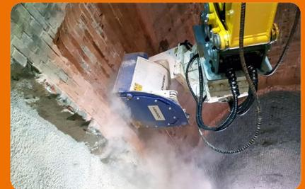
Productivity meets accuracy: the mechanical or hydraulic depth control assures a constant cutting depth while working with the KEMROC attachment.
