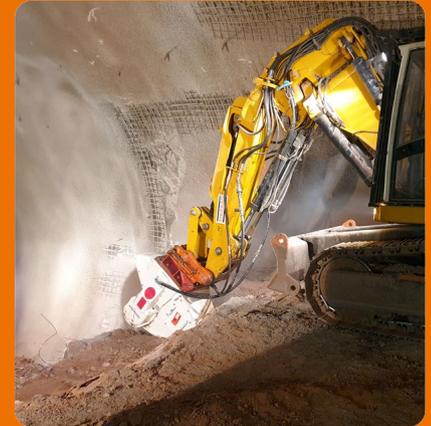
The HOCHTIEF / Züblin contractor demolishing a temporary tunnel invert support made from shotcrete using a KEMROC cutter wheel in the Trimberg Tunnel.
