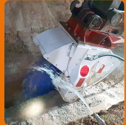
The cutter wheel in close-up. The DMW 130 cutting wheel achieves a cutting rate of around 15 – 20 m/h in shotcrete.
