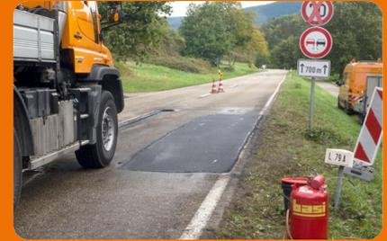
Repair of the road section near the town of Gernsbach is finished. After a short period of time to allow the asphalt to cool, the road is opened for traffic.
