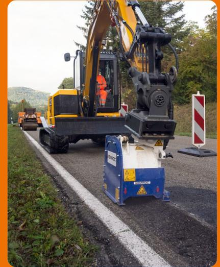
A KEMROC EX 30 HD patch planer mounted on a 6-ton excavator used by the Gernsbach road maintenance department to remove asphalt from damaged sections of roadway.
