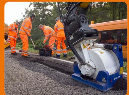
The KEMROC EX 30 HD has stepless and precise depth control. At this location, a 4 cm deep layer of asphalt is being removed.
