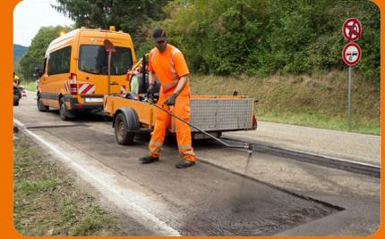
After removal of the damaged road surface, the surface is sprayed with a bitumen emulsion, ensuring permanent adhesion for the new road surface layer.
