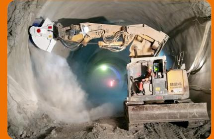
A KEMROC DMW 130 cutter wheel was used to cut slots in the outer lining of the Cannstatt railway tunnel for the installation of drainage channels either side of dam rings. They are needed to protect adjacent anhydrite deposits from groundwater ingress.
