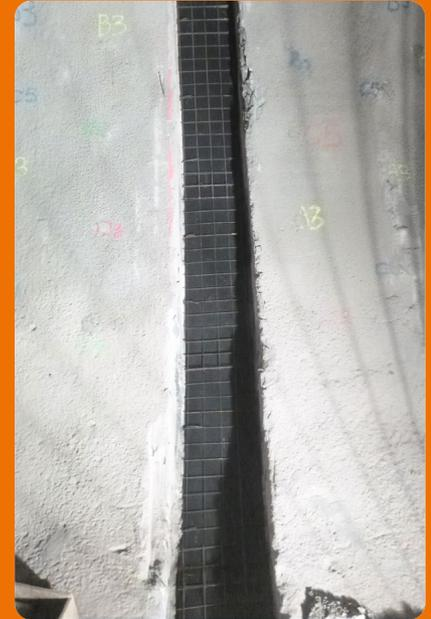
An unusual application for the KEMROC cutter wheel resulted in a surprisingly high speed rate. The minimum amount of material was excavated, reducing the amount of shotcrete required to fill the void in the tunnel lining.
