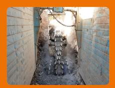
In contrast to the use of a conventional drum cutter, it isn't necessary to slew the excavator arm and attachment during operation. This makes it easier to work between trench supports; a major advantage when working in ground that is not homogenous.
