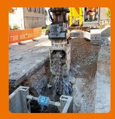
While trenching at Steinsfeld in central Franconia, the experienced contractor LEONHARD WEISS meets deposits of gypsum. In these conditions it paid to use a KEMROC chain cutter attachment on a 32-ton excavator.
