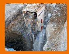
The chain cutter excavates a trench with the required profile to the required depth. This reduces the amount of material cut and the amount required for backfill which also keeps transport costs to a minimum.
