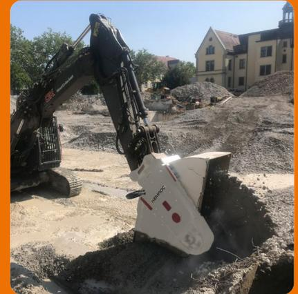
At a project in Konstanz, CK Abbruch & Erdbau GmbH had to break up a huge concrete pad. The trial rental of a KEMROC cutter wheel was so successful that the company purchased an identical machine.
