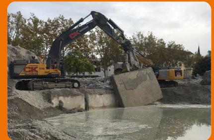
The demolition method involved cutting out 15 m<sup>2</sup> blocks which were subsequently lifted out using an 80-ton excavator.
