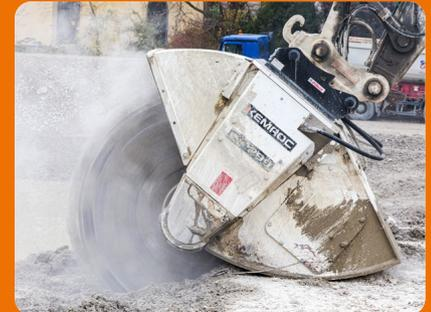
The cutter wheel purchased by CK Abbruch & Erdbau in action. The operator cuts through the 10 cm thick concrete slab at a speed of 10 – 15 m per hour.
