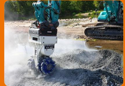
The KEMROC drum cutter was mounted on a 26-ton Kobelco SK 280.
