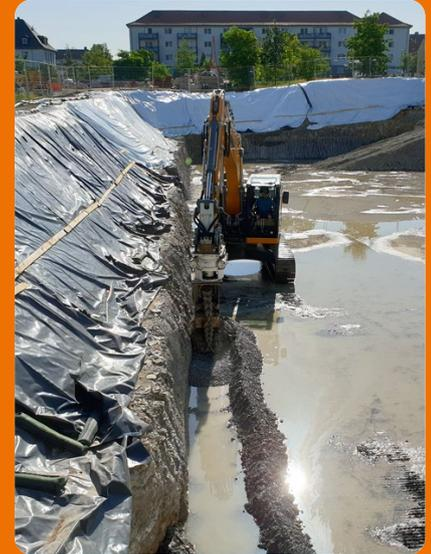
In contrast to the use of a breaker, the sudden build-up of rainwater or standing water in the trench has no adverse effect on the operation of a cutter. On the contrary, it makes the cutting process easier.
