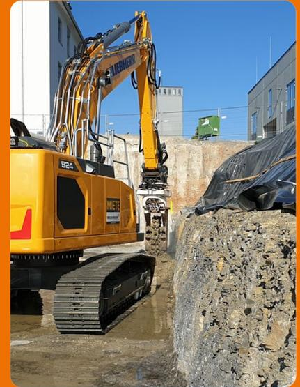
With a rotation module between the excavator arm and cutter attachment the operator can excavate the trench parallel to the side wall regardless of the position of the excavator. This also avoids excavating a larger trench than necessary.
