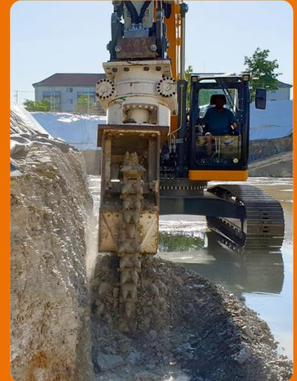
The construction company Höhn had to excavate a drainage trench at the job site of the State Fire Brigade School in Würzburg. The combination of a 24-ton excavator with KEMROC EK 100 chain cutter proved to be ideal for the project.
