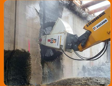
A KEMROC cutter wheel is then used to cut through the last 100 cm of the wall. A second cut frees up a segment of the tunnel lining.
