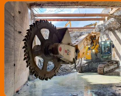
Partial demolition of a tram tunnel in Stuttgart. The photo shows a tunnel excavator with a KEMROC cutter wheel attachment.
