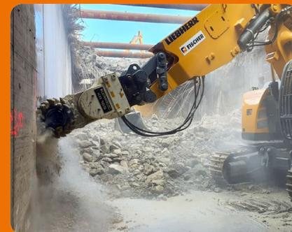
The first step is to reduce the thickness of the tunnel lining to about 100 cm using a KEMROC rotary drum cutter.
