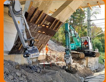
Using more machines reduced labour costs. For this project two excavators fitted with KEMROC drum cutters rented from TBH were used.
