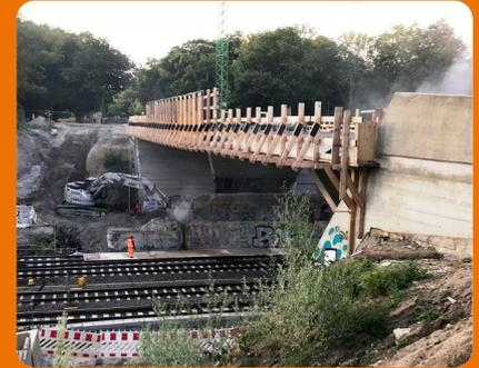
The new Messebrücke in Leipzig is a bridge spanning four railway tracks. The pillars of the original bridge were demolished after the new replacement bridge had been constructed.
