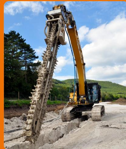
Before cutting into the ground, the full length of the sword is visible. For the first phase of the installation of a diaphragm wall at the retention basin a KSI 5000 attachment with 5 m long sword is used mounted on a 50-t excavator.
