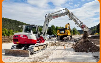
An eight-ton excavator prepares the site for the larger excavator fitted with the KSI mixing attachment. Removing some surface material along the line of the diaphragm wall prevents binder solution with cement from flowing away from the working area.
