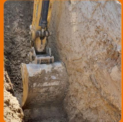
At various distances along the length of the hardened diaphragm wall, sections are exposed using an excavator. Tests indicate that the soil cement structure has the required shape and density necessary for this flood protection project.
