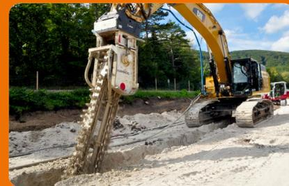
Mixing and stabilising soil by the addition of a cement suspension in a binding agent – using the KSI injection attachment from KEMROC, stable soil cement structures can be created in-situ. Engineers at PORR used the attachment when constructing a retention basin in Pottenstein (Lower Austria).
