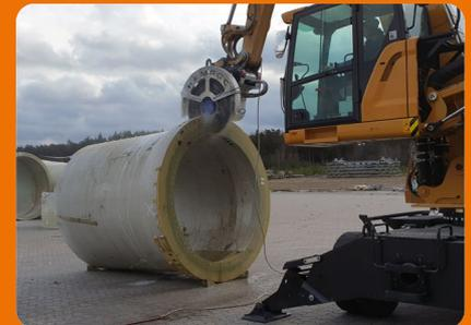
The hydraulically driven diamond saw is used to cut the rotor blades into smaller sections.
