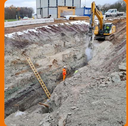
A sub-section of the A3 autobahn upgrade project in northern Bavaria. Drainage pipe trenches were excavated on site at the Steigerwald service area.
