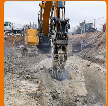
Civil engineering company BUNTE rented a 42-ton excavator with a KEMROC EK 150 chain cutter to excavate trenches in the bedrock.
