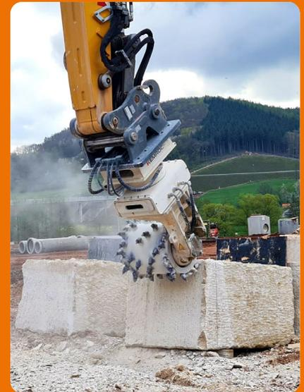
The portal walls are clad with massive Jurassic limestone blocks. Pre-cut blocks were delivered on site and then they were ground to the exact length.
