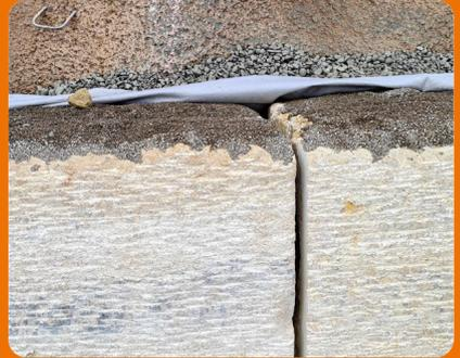
Two of the 9,000 blocks used to clad the walls. Due to being ground accurately to length, the STRABAG specialists can maintain the required joint tolerances.
