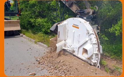
Engineers from Bautechnik Schödl use a KEMROC SMW 80 cutter wheel to excavate trenches for fiber optic broadband in Schneeberg.
