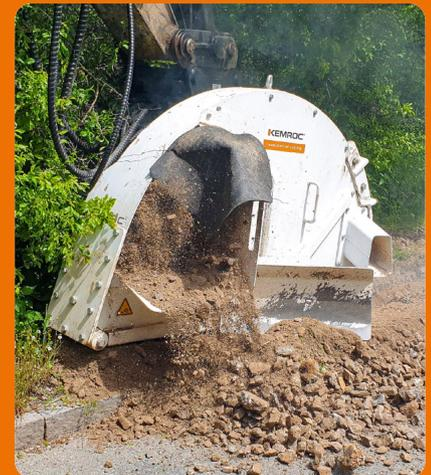
In one operation, the cutter wheel excavates a trench in overburden with rock or through asphalt while depositing the spoil along the side of the trench.
