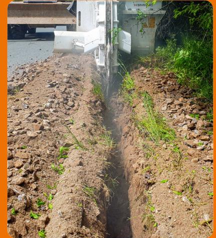
The exposed trench is ready to take the empty conduit which is protected by a layer of sand and the filled and compacted.
