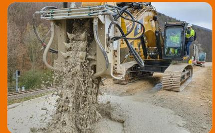
The cutter chain penetrates into the ground and mixes it with a binder suspension fluid from a semi-mobile mixing plant. After hardening, a homogenous, dense, load bearing soil-cement structure is created.
