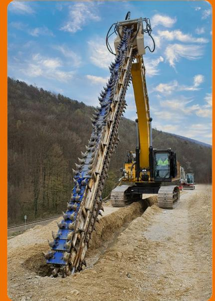
KEMSOLID is the name of the KEMROC's process for soil stabilisation and ground improvement. A central element is the KSI mixer attachment mounted on a standard excavator.
